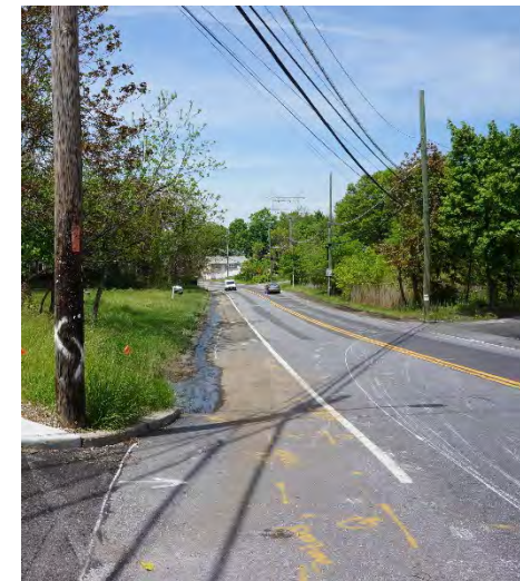
Figure 27: Excessive shoulders in certain locations could be utilized to reconfigure road alignments to include left turn lanes or center medians.
