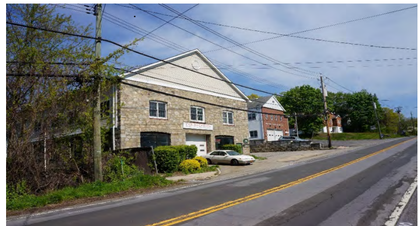
Figure 10: Parallel and perpendicular roof ridges add to the attractiveness of the Village
