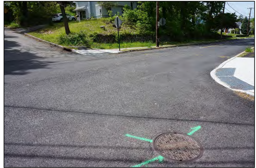
Figure 19: The intersection of Albany Post Road, Lindsey Avenue, and Gallagher Street is an example of where crosswalks and traffic calming measures could ease the conflict between pedestrian and vehicle traffic
