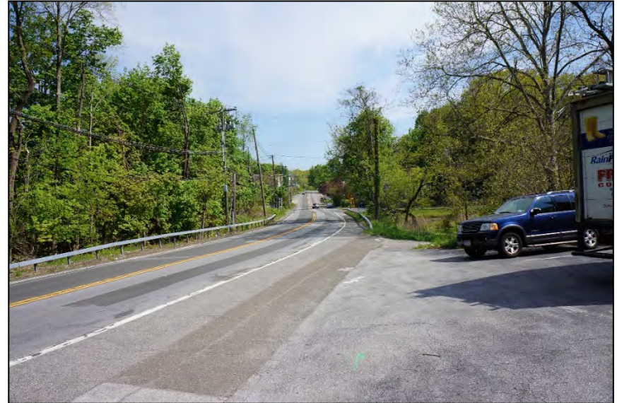
Figure 25: A route devoid of pedestrian amenities becomes uninviting to pedestrians. Also, a continuous driveway illustrates poor access management and creates potential traffic conflicts.
