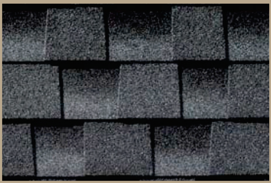
ROOF ASPHALT SHINGLE
