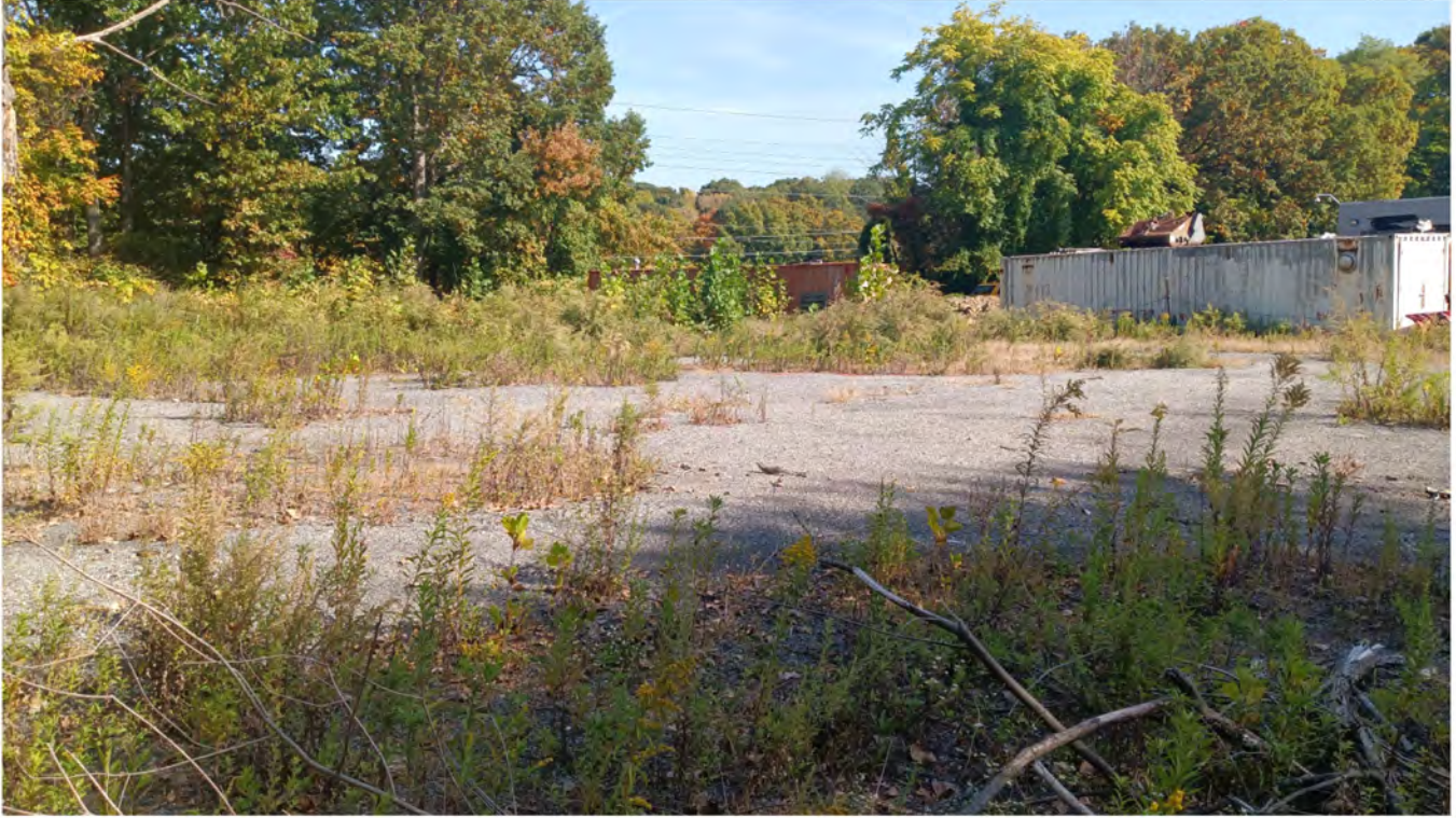
Existing pavement in area of proposed stormwater wetland
