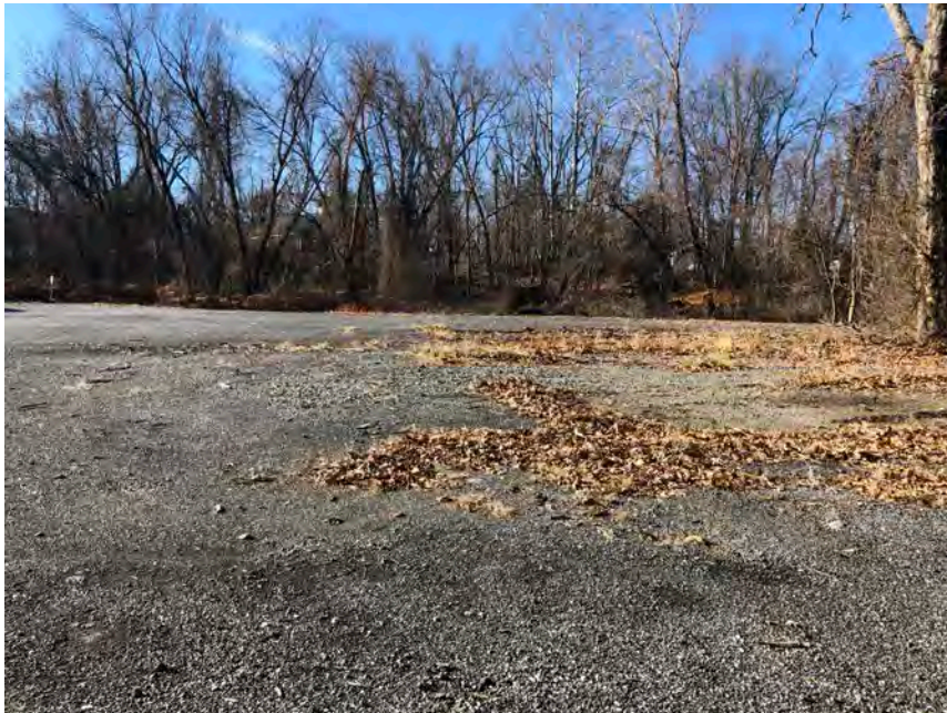
4. Gravel area, eastern-central portion of property
